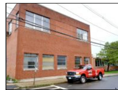
Demolition less than expected
